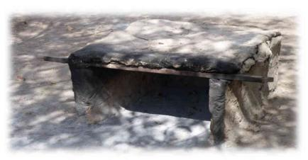
STEP 2: build a 3-walled structure, using bricks and cement, with bricks overlapping for solidity, as shown. It shouldn't be too high, 50cm at most, in order to retain heat. Leave to dry completely.
